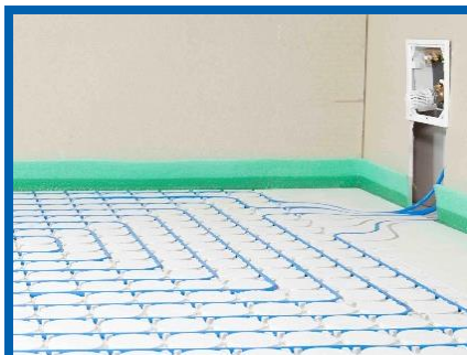
FLEXIRO dry-lined underfloor heating, laying pattern: meandering
